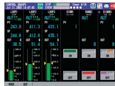
DIO operation monitor screen
